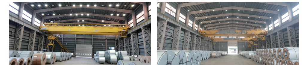
► Before installing LED lights
